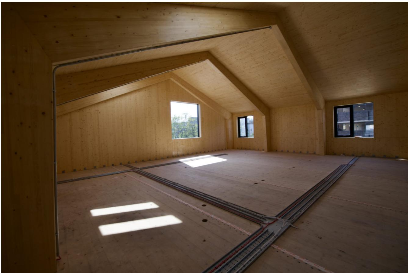
The existing building has been largely retained and sensitively refurbished while the extension is built with a Glulam frame and CLT (cross-laminated timber) wall panels with zinc wall- and roof-cladding. Polyester powder-coated aluminium glazing and curtain-walling elements are used throughout as a unifying element for the two parts – old and new – that make up the extended building.
